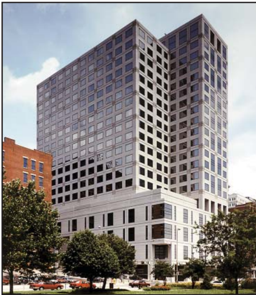
Standard Insurance renewed its lease at Duke Realty's 312 Plum Building, who provided an additional 18,000 square feet of expansion space at 312 Elm (above).
